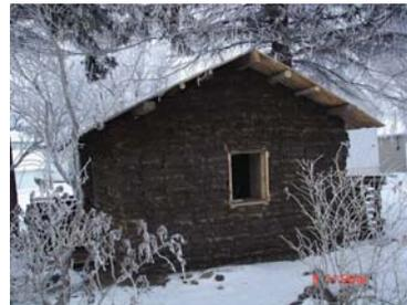
one would lay bricks, locking the rows together. The window and door frames were constructed and placed as the walls went up. Sod was stuffed around the frames for added insulation. The sleeping loft was added to stabilize the walls as well as to add more living space to the small structure. The door was constructed of 1-inch rough oak boards with Z-bracing and 4-pane barn windows finishing the room. The soddy was erected under huge pine trees to keep minimize wind and water erosion.
