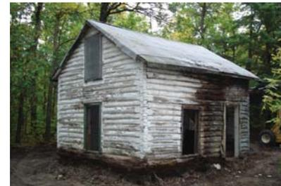
was in overall good condition, mainly because it was constructed of tamarack logs. However, the bottom three rows of logs were in poor condition due to the addition of a poured concrete retaining wall that was meant to keep out rodents. Moisture and leaves became trapped in the wall causing severe deterioration of the logs. Windows, curtains, and some furniture from the previous owner remained in the cabin.
